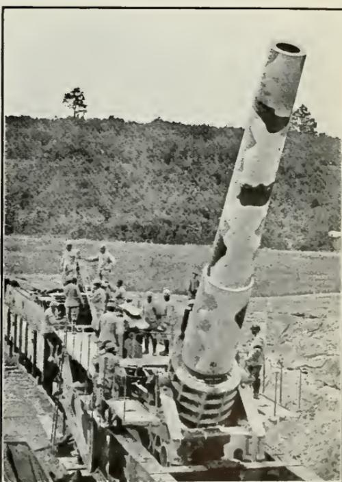
Big gun, *camouflaged*, mounted on railway truck.
