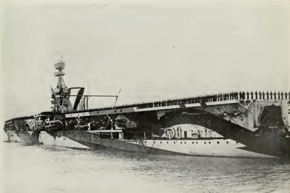
The British ship *Furious*, a "hush" cruiser, "dazzle" painted, used as a floating aërodrome. *The ship is covered with a long, broad platform upon which the aëroplanes start and alight.*
